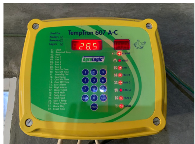
Gambar 22. Micro-climate control tipe TempTron 607 (Dok. Penulis, 2023)
